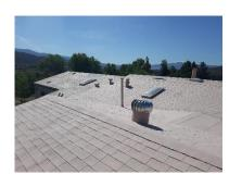
ACS CIC 4.0 was applied on top of asphalt shingles to block solar heat loading
